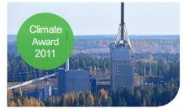
World's largest Waste-to-Energy Gasification Plant, Lahti Energia
