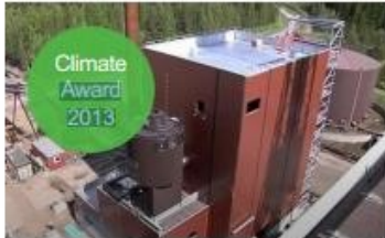
First demonstration scale integrated pyrolysis unit, Fortum
