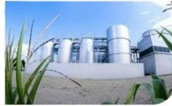
Germany's largest lignocellulosic ethanol demonstration plant, Clariant
